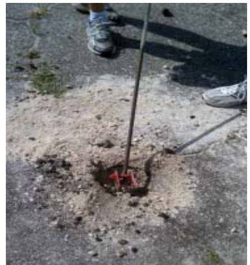
Finished tie down!
